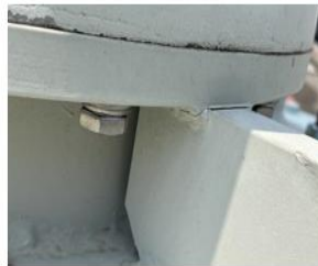
Crack observed on HV Bushings Flange
